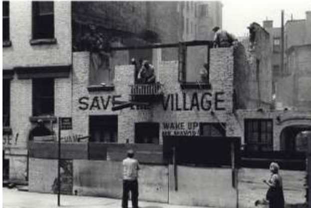
Fred W. McDarragh, "Demolition of Artist's Studio, Greenwich Avenue, May 19, 1960"
